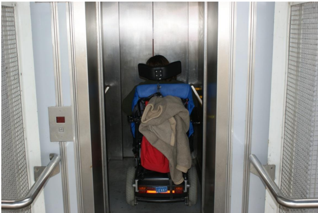
Figure 6: participant in motorised wheelchair in the lift at Greenwich DLR (control panel is to the immediate right of the participant), this participant had an assistant who travelled with them, who only just fitted in the lift at the same time.
